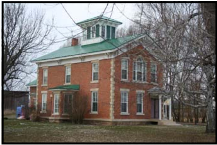
#2—Arial P. Rublee House, circa 1860's., N4785 CTH M, Town of Hamilton. This two story Italianate style residence has a gabled roof with a prominent cupola.
