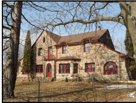
#2—John and Razy Wright House, 1924. This romantic style pseudo Tudor home is located at W5670 CTH F in the Town of Medary. Its unique Flemish Bond stone exterior, and arched windows and doorways were designed for the Wrights by regional architect Otto A. Merman.
